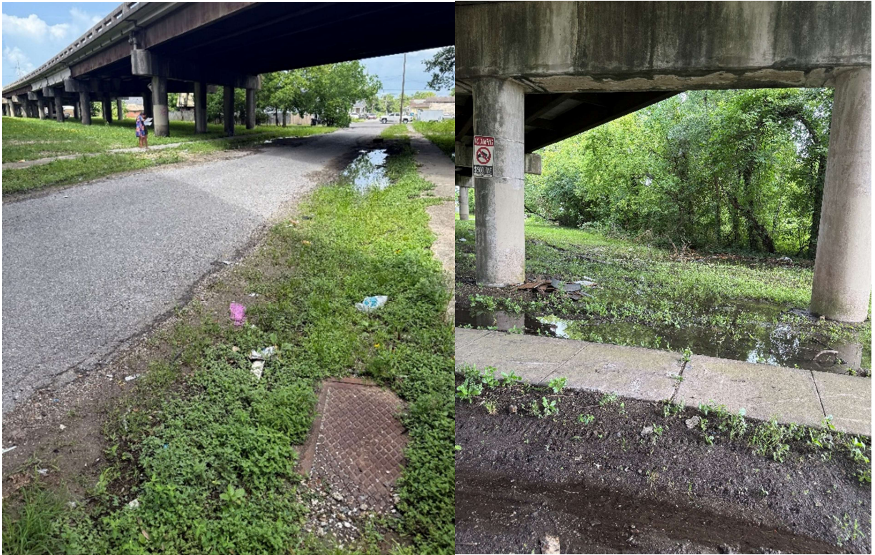
Figure 9: Flooding and Clogged CB Under I-10 at N. Johnson St
