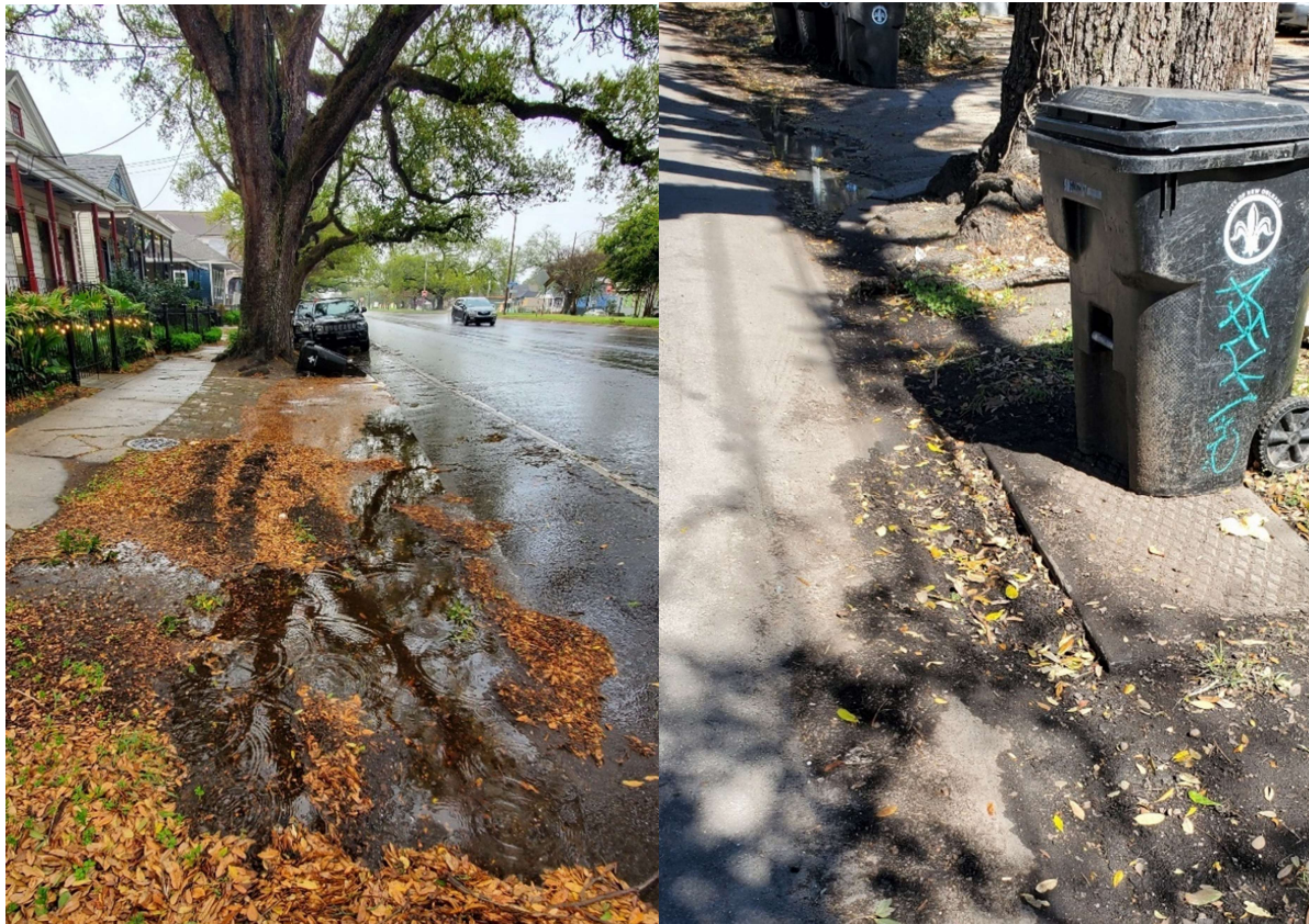
Figure 21: Evidence of Leaves and Clogged Catch Basin on 1900 Elysian Fields
