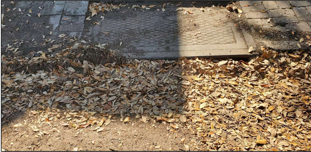
Figure 12: Blocked Catch Basin on 1800 Elysian Fields Ave
