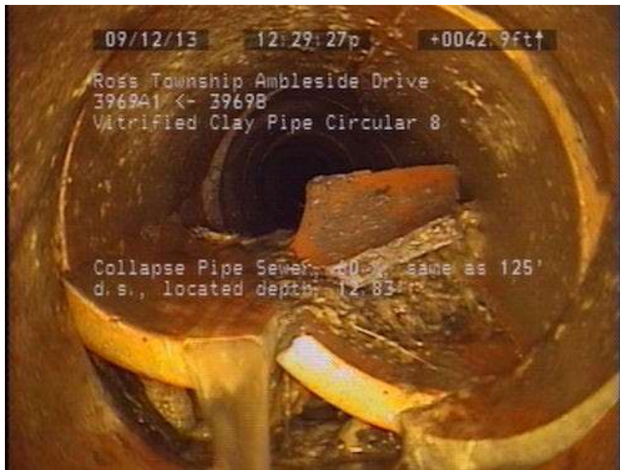
Figure 9: Example of Broken Terracotta Drain Line
