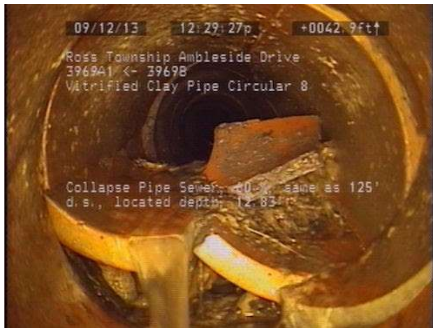
Figure 8: Example of Broken Terracotta Drain Line
