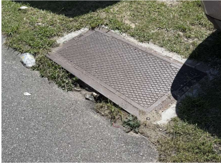
Figure 10: Sunken Catch Basin on 900 N. Tonti St
