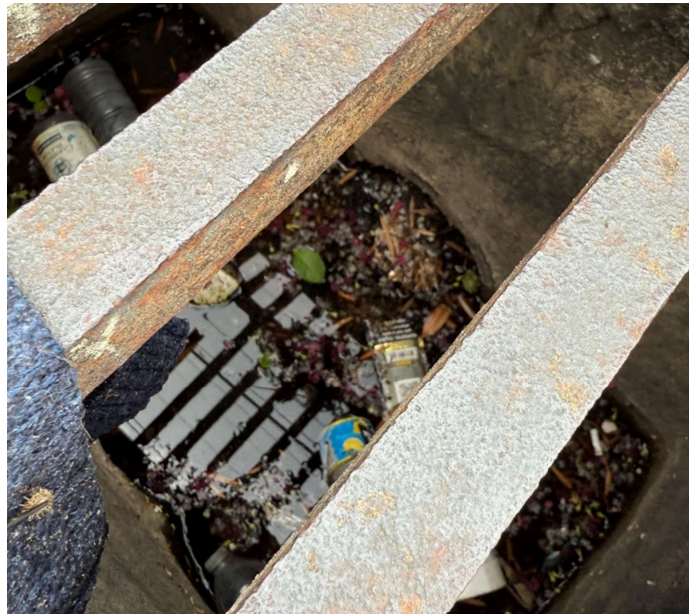
Figure 12: Visual Evidence of Blocked Inlet on 800 N. Prieur Street
