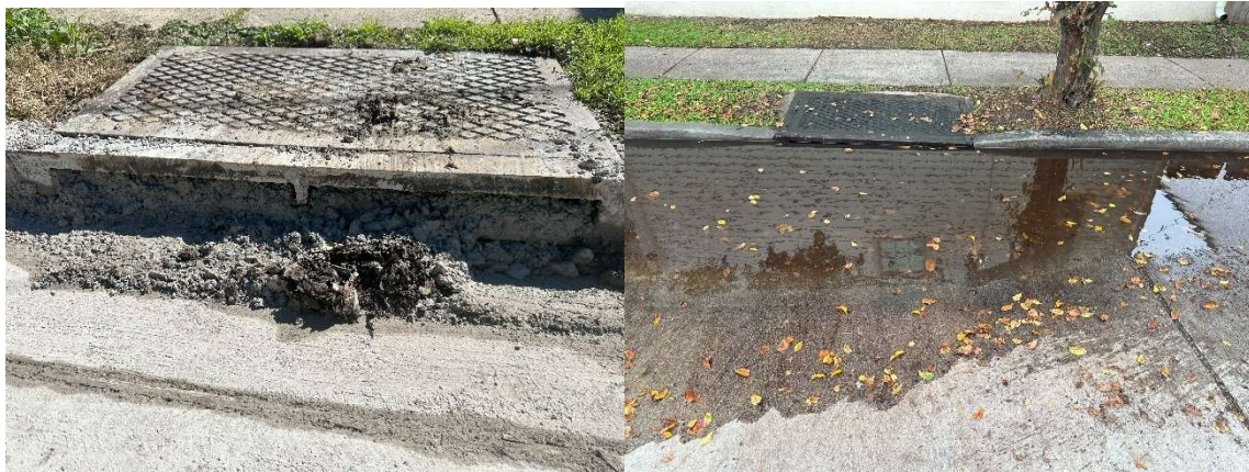
Figure 19: Resident Photos: Non-Functioning Catch Basins on 1500 Dumaine and 900 N. Robertson, respectively
